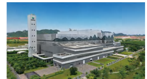
Nanning Shuangding Circular Economy Industrial Park Project
